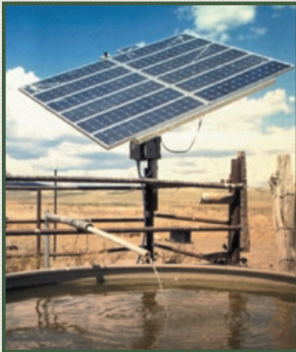
Ute Mountain Indian Reservation solar water pumping
