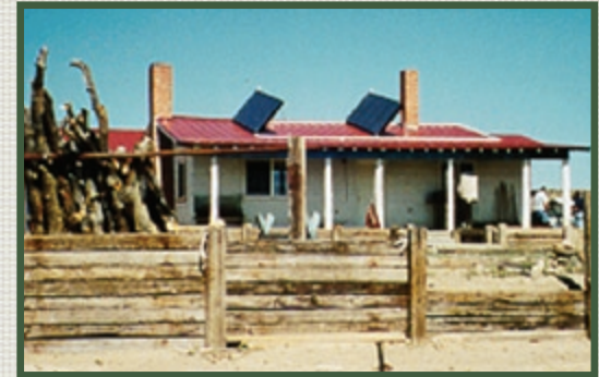
Solar installation at Pueblo of Laguna's Majors Ranch.
