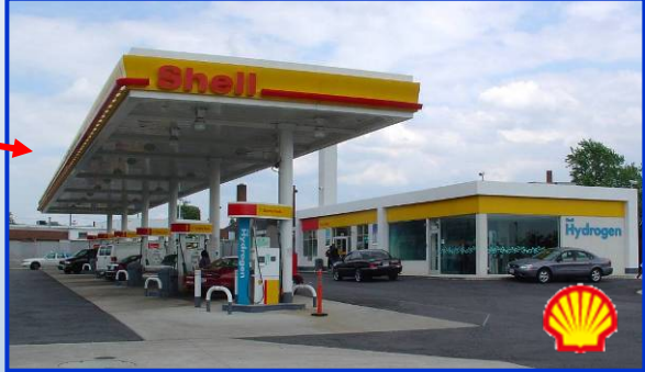
Hydrogen and gasoline station Washington, DC
