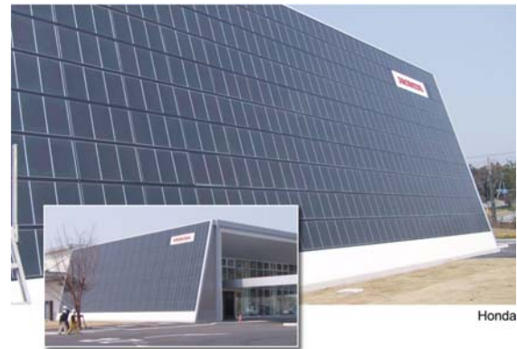
Figure 5: Building-integrated thin-film CIGS façade on a Honda building in Japan
