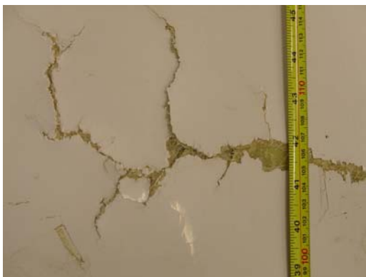
Figure 24: Crack near blade centerline on TX-100 blade.
