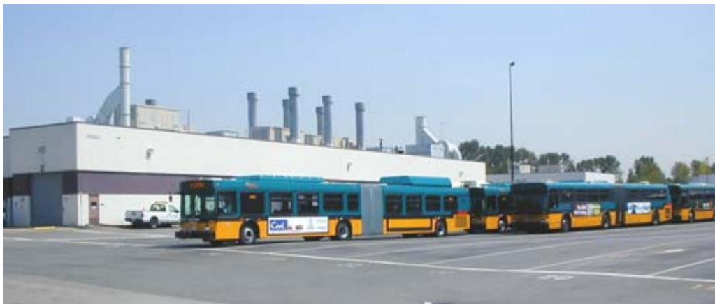
Figure 10. South Base Maintenance and Office Building
