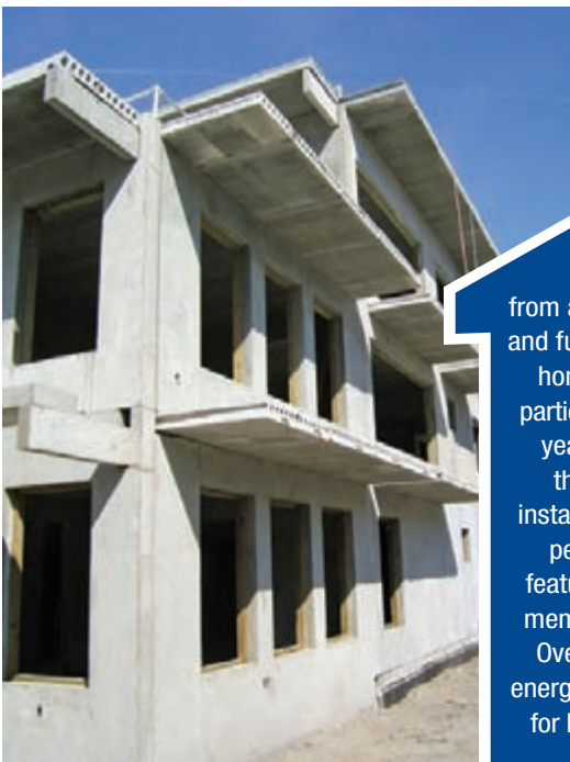
Pre-cast concrete overhangs provide area for vegetation and shade to reduce solar heat gain.
