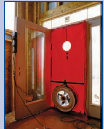
Home airtightness is tested with a blower door.
