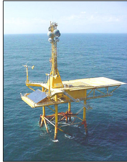
Figure 4. Pictures of the Savannah Light Station (left) and U.S. Navy R2 Tower (right)
