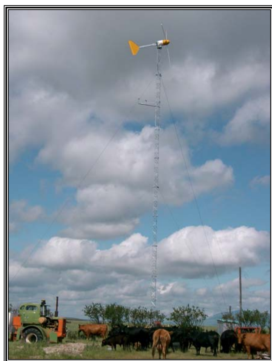
Tower type/height: 30m standard guyed. Commission date October 8, 2003. Host site: Jess Alger.
