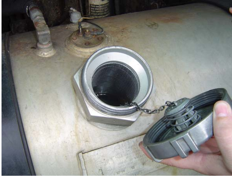
Figure 9. Flame arrester in place on refuse hauler fuel tank at E.J. Harrison & Sons
