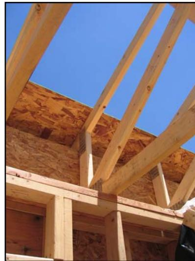
Fig. 4: Raised heel trusses
