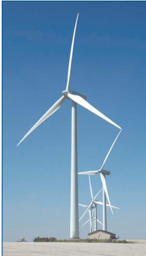
The Kumeyaay Wind Power Project is comprised of 25 Gamesa 2-MW turbines.
