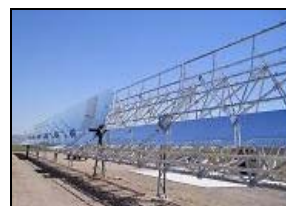
Fig.1 . Deployment of advanced trough structure.
