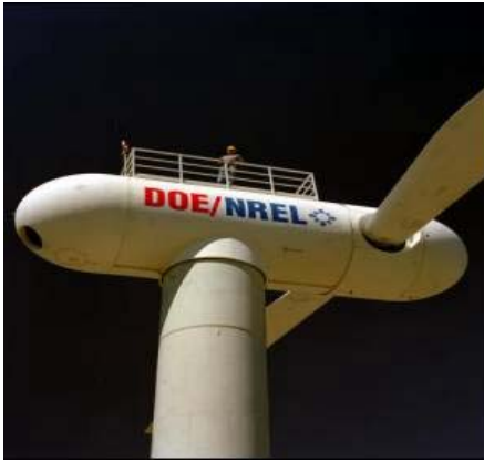
Figure 1. The Controls Advanced Research Turbine (CART).
