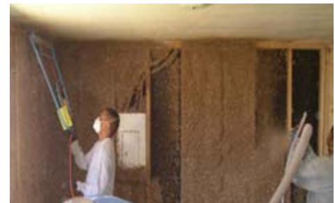
Figure 8. Blown Cellulose Insulation
