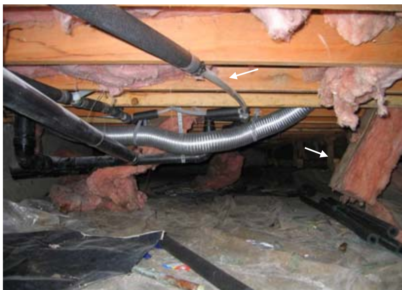
Figure 14. Crawlspace of Unit #303
