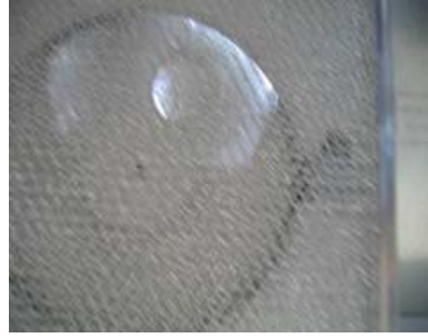
Figure 7. Looking up kitchen exhaust
