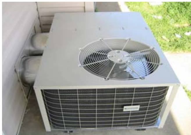
Figure 9. Packaged heat pump unit for house #303
