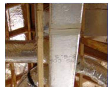
Mastic provides the most reliable duct sealing method for new construction.
