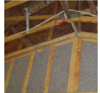
Blown-in wall insulation
