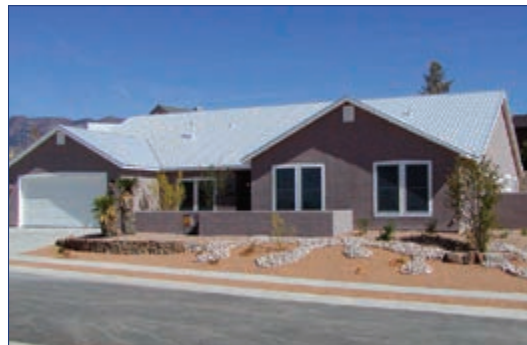
Artistic Homes of Albuquerque New Mexico built 650 homes in 2003, all of them using Building America principles.
