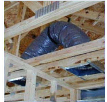
FIGURE 19: Jump Ducts
