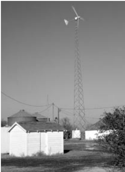
Warren Gretz, NREL/PTW09634
