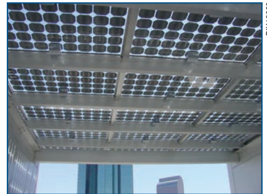
Building-integrated PV is located along the roof of the building. The PV cells are sandwiched in translucent glass panels and mounted horizontally to form seven shaded bays at the penthouse level.
