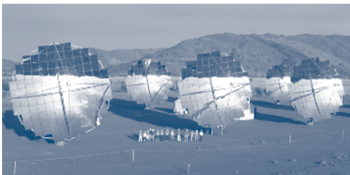
Figure 6. These 20-kW Solar Systems dishes dwarf visitors in Alice Springs, Australia. The concentrators use an array of mirrors to focus sunlight onto high-efficiency cells. Four supports hold the cells in front of the mirrors; the supports also supply cooling water and electrical connections.
