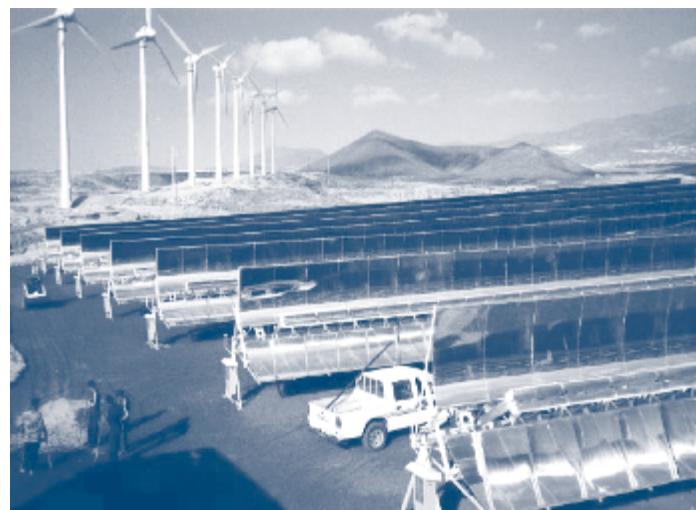
Figure 1. Parabolic troughs, like those used in this Euclides-Thermie installation in Spain, concentrate sunlight onto a strip of high-efficiency solar cells positioned above the troughs.
