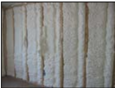
Spray foam insulation
