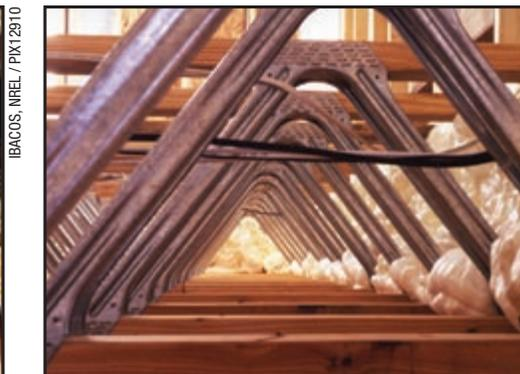
Open web trusses provide space within the building enclosure to run electrical wires and ducts.
