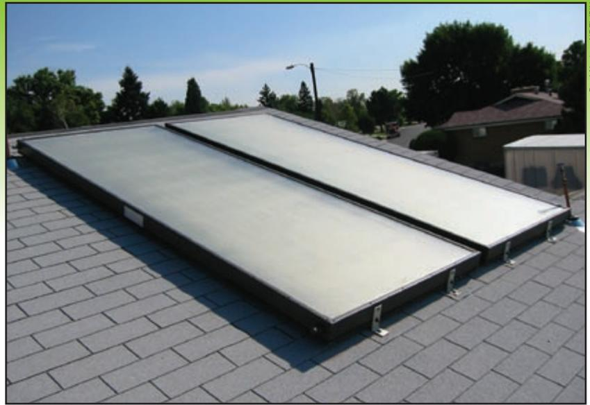
Solar water-heating collectors
