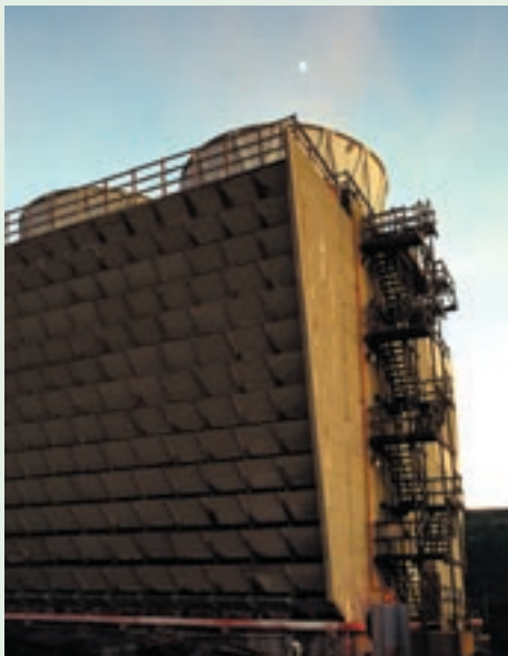
Geothermal power plants use cooling towers, like these at The Geysers, to safely reject waste heat into the atmosphere.
