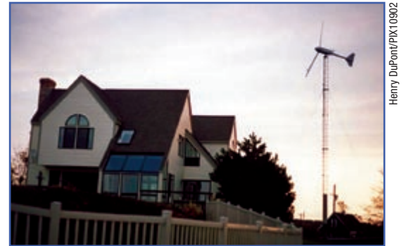
Figure 9. The Bergey Excel 10-kW wind turbine at the Evans Residence, Block Island, Rhode Island.
