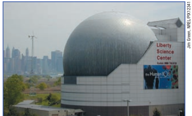
Figure 10. The Bergey Excel 10-kW wind turbine at the Liberty Science Center in New Jersey helps reduce the Center's electricity bill and feeds excess power to the utility grid.
