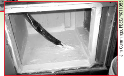
Repair of a platform return. Before (top): Note the cracks and gaps along the edges and joints. After (right): The same platform return after it has been sealed from the inside using mastic.
