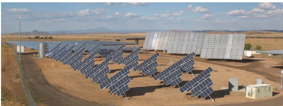
Figure 2. Photograph of field of PV systems at APS' Prescott, AZ, facility. The three large (35-kW) CPV systems on the right are Amonix systems. The systems on the left are single-axis-tracking, flat-plate silicon systems.
