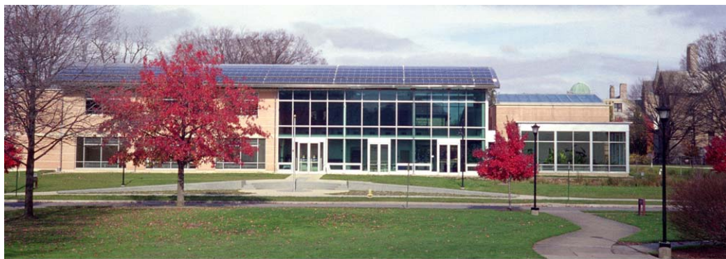
Figure 1. Oberlin South Facade Showing the PV Array on the Roof
