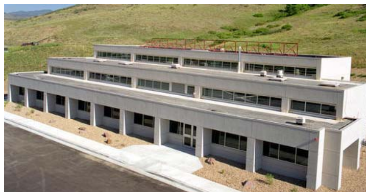
Figure 4. NREL Thermal Test Facility
