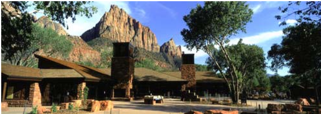
Figure 2. Zion Visitor Center North Elevation Showing Cooltowers and Plaza
