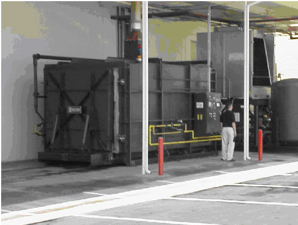
Figure 7. Furnace for reactor mockup work.
