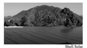
Figure 7: 245-kW rooftop, thin-film CIS-based solar electric array, Camarillo, California
