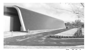
Shell Solar Figure 6: 85-kW thin-film CIS-based BIPV facade, North Wales, UK
