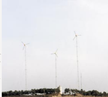
Four Bergey Excel 10-kilowatt wind turbines in Xiao Qing Dao Island village.
