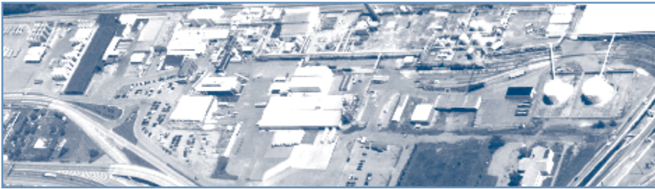
Rohm and Haas' Knoxville, Tennessee plant
