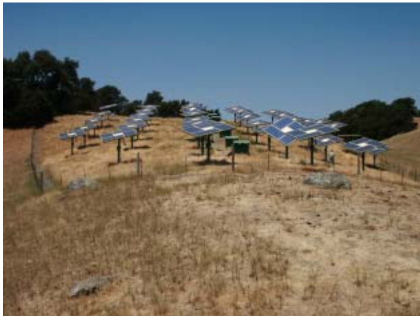
Figure 30: Array of 144 MSX 240 Modules on Trackers in California
