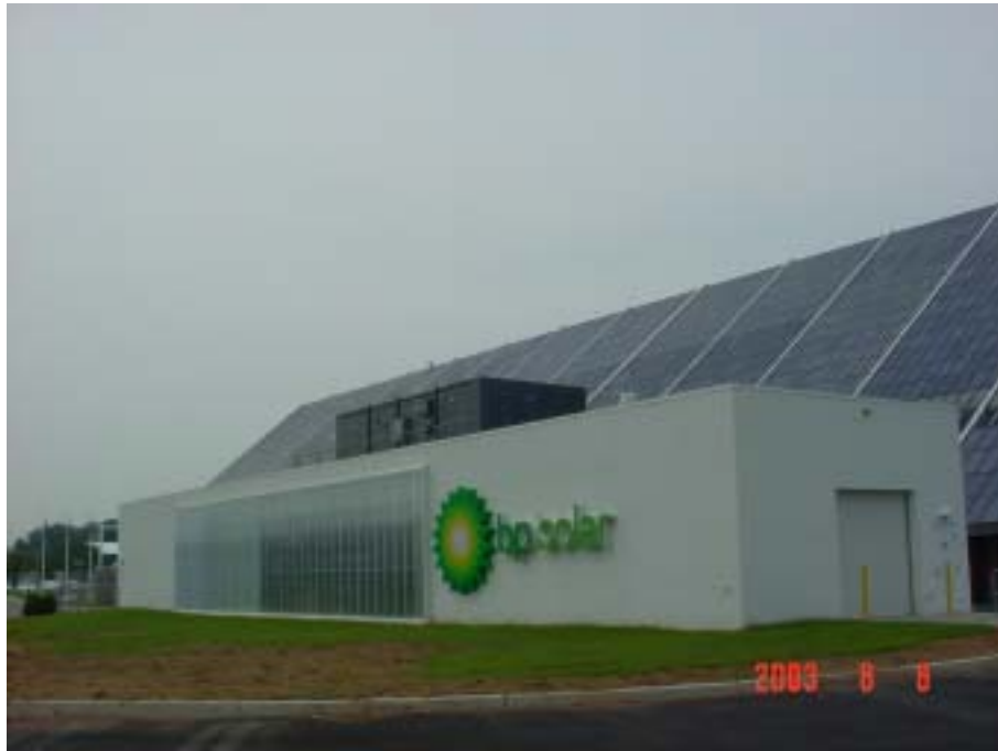
Figure 25: New Building for Silicon Nitride Deposition – Frederick
