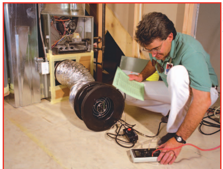
Building America researchers analyze the whole-house energy performance of newly constructed homes by conducting different types of field tests. In this photo, a Building America staff member performs a duct blaster test to measure the impact of duct leakage on whole-house performance.
