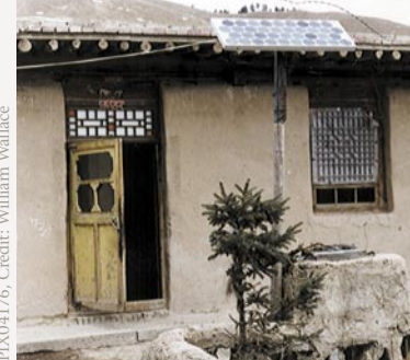
Solar home system in Gansu Province, People's Republic of China.
