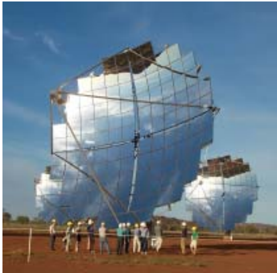
Figure 1: Solar System concentrator PV unit with one receiver on each unit.
