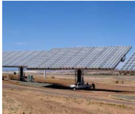
Figure 2: Amonix concentrator PV unit with seven receivers.
