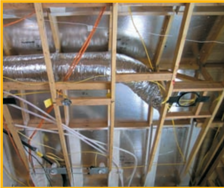
A radiant barrier prevents the sun's heat from seeping into the attic. Ducts are sealed and insulated.
