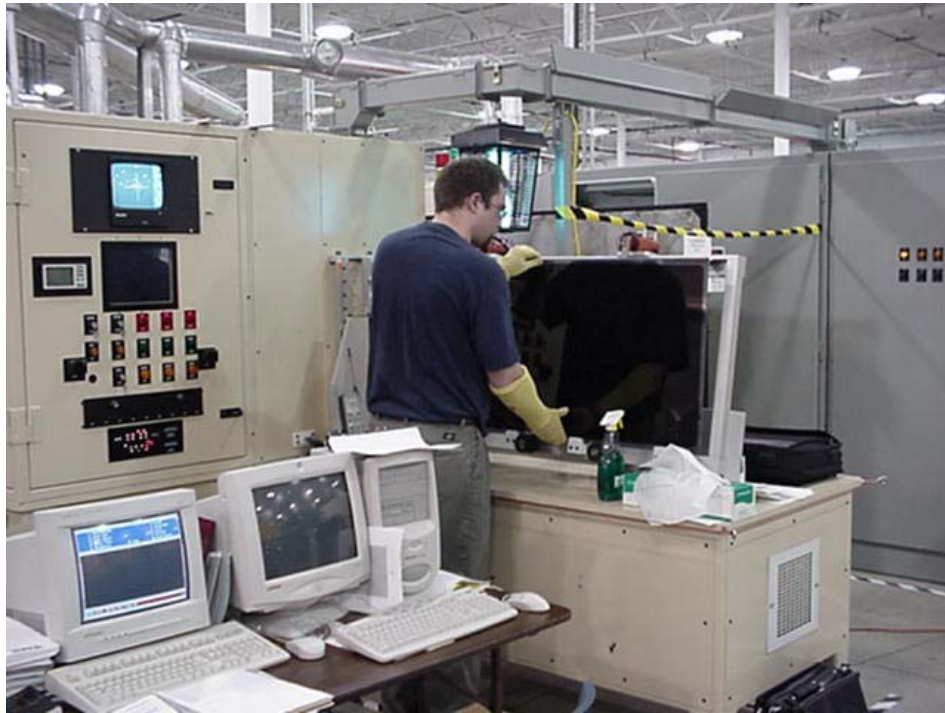
Figure 12. Photograph of First Solar rapid laser-scribing system, showing the loading station, the process control station the scribing station (enclosed in cabinet), and the power-supply station (to the rear)
