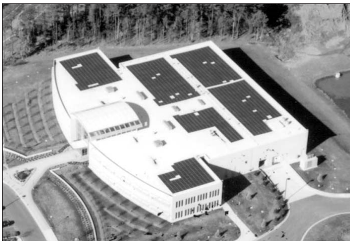
The Environmental Protection Agency's new facility at Research Triangle Park, North Carolina, was designed to be energy efficient and to produce electricity on site by means of a rooftop photovoltaic (solar electric) system.
