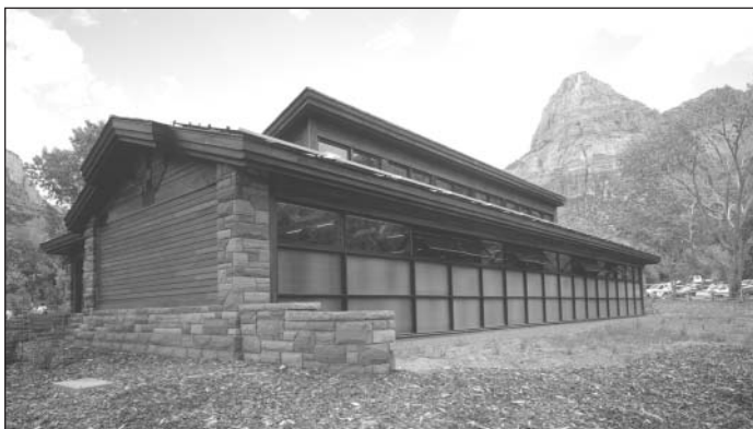
The Zion National Park Visitor Center in southern Utah was designed to be a model of sustainability, incorporating the area's beautiful natural features as well as numerous elements that save energy and reduce operating expenses; the center also features a photovoltaic system for on-site power generation and a Trombe wall for solar heating.
