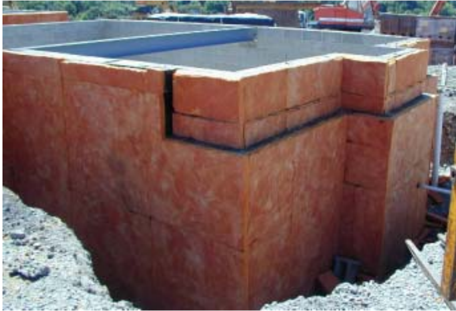
Figure 1. The semi-rigid fiberglass board insulation, 2-3/8 in. thick, provides R-10 thermal performance and water drainage at the exterior of the foundation wall. It was applied over a dampproof coating to the height of the sill plate. The exterior edge of the brick or wall sheathing above the board was designed and installed so that the edge would lay flush with the foundation wall, thereby protecting the top edge of the insulation board.
