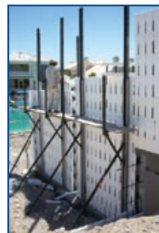
Steel beams (left) for structural framing are anchored into the insulated concrete form wall, and (right) insulated concrete forms make up the exterior shell of the home.
