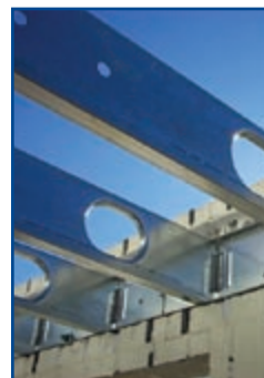
Steel beams (left) for structural framing are anchored into the insulated concrete form wall, and (right) insulated concrete forms make up the exterior shell of the home.
