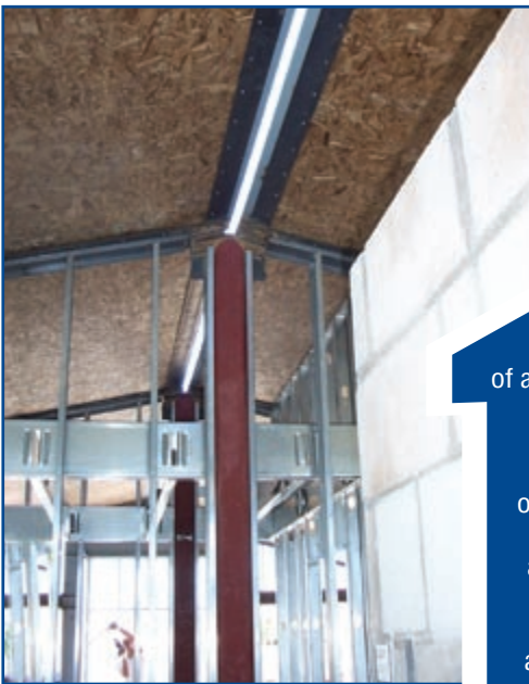
Structural insulated panels provide the air and thermal barrier for the roof.
