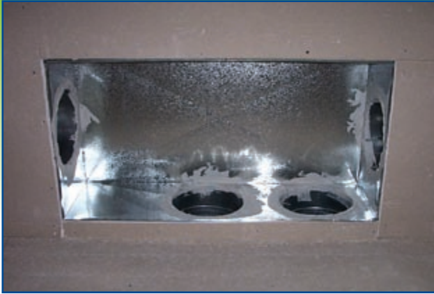
UL-181 approved mastic properly seals the entire duct system.
