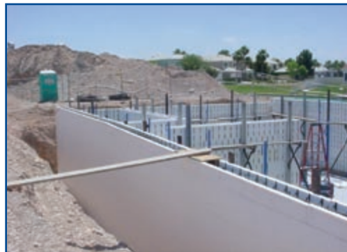
Insulated concrete forms form the walls of the basement.
