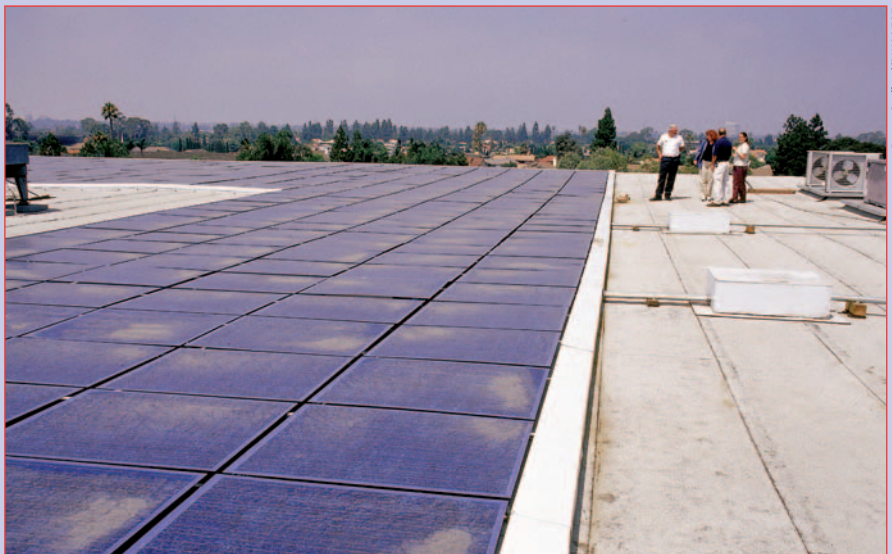
Arden Realty of Fountain Valley, California, uses this 240-kW solar electric system for its company headquarters.
