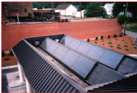
The Central Carolina Bank, Bessemer City, North Carolina, uses a 2.75-kW solar electric system to produce electricity and heat for this building.
