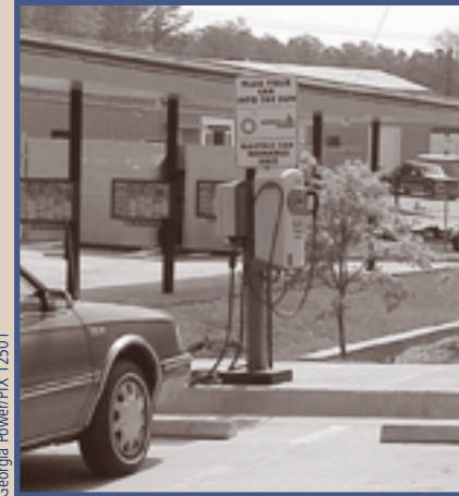
"Plug in the Sun" stations feed current to EVs and to Atlanta's power grid.
