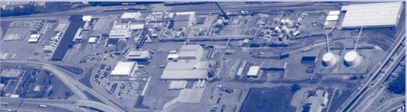
Rohm and Haas' Knoxville Plant
