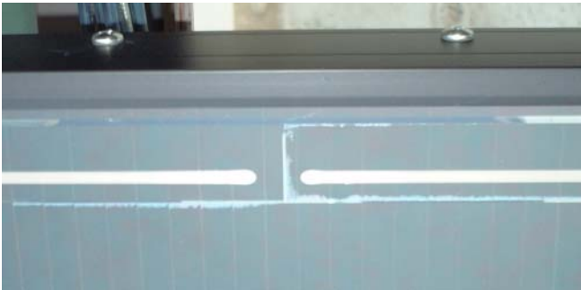
Figure 6. A photograph of the front surface of an a-Si module installed in a 1-kW PV system at NREL for about 3 years.
