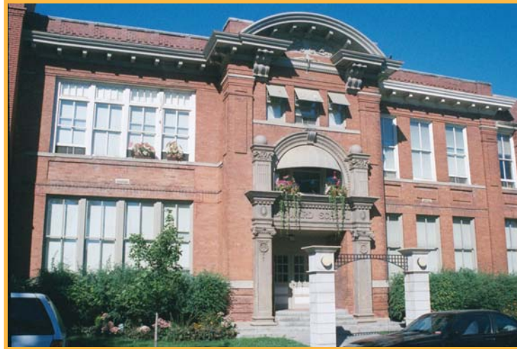
Seventy-one windows were replaced in Lincoln's oldest surviving school building, now Hayward Place Condominiums.
