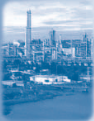
A California refinery's plant-wide assessment identifies $52.5 million in energy savings. See page 6.
