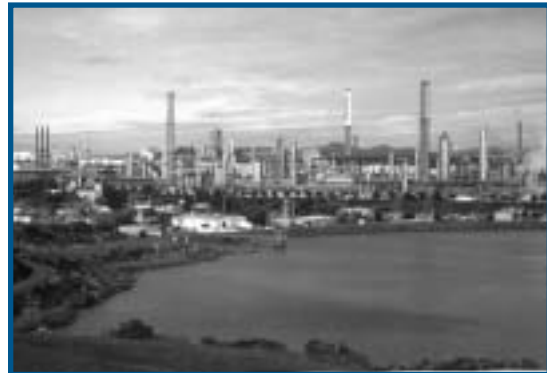
The Martinez Refinery was the focus of a plant-wide energy assessment.
