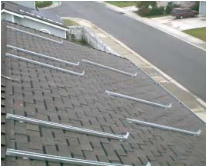
Figure 10. Final Design – Runners Attached to Roof
