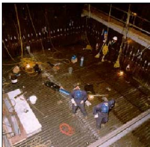
Figure 11: Routine Maintenance Inside of a Boiler 35
