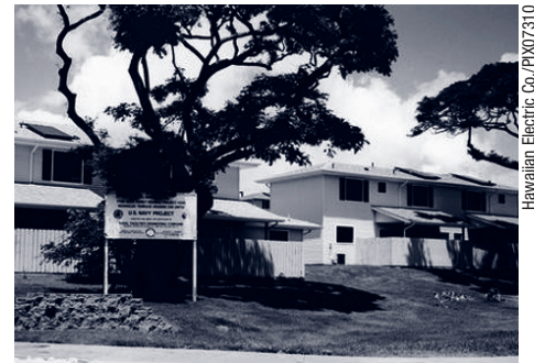
At the Navy’s Moanalua Terrace housing complex in Hawaii, 366 rooftop solar water-heating systems offset about 622 tons of carbon dioxide emissions each year.
