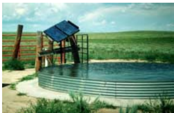
Figure 2.2. A water storage system for cattle watering using a PV pumping system.
