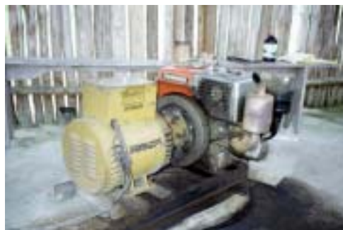
Figure 3.1. Diesel generator at a rural Panamanian hospital.
