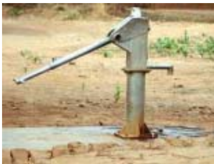
Figure 4.2. An Indian Mark II-type hand pump used in rural villages.
