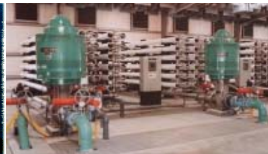
(d) Large RO water purification plant (four each a million gal/d capacity). Courtesy of American Engineering Services Inc.
