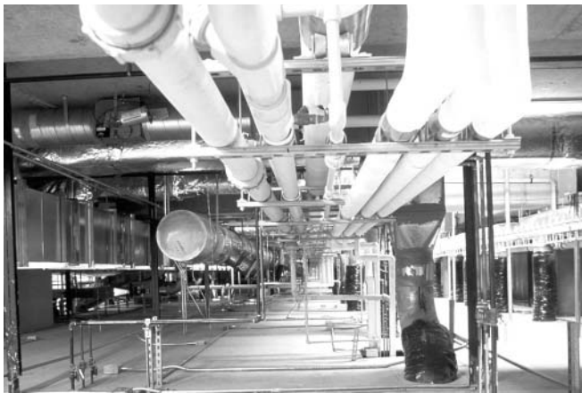
Interior view showing interstitial space.
