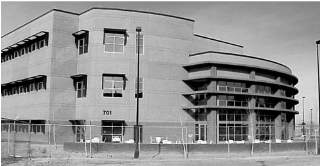
Sunshades protect windows from the hot summer sun.
